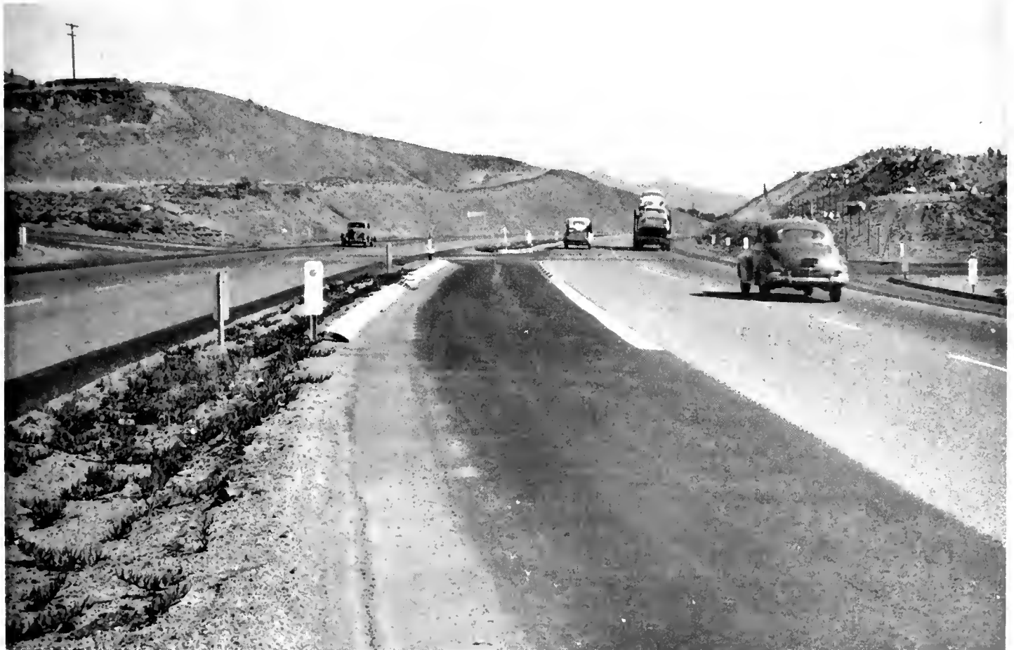
Sign Route 78 between Oceanside and Vista. Typical intersection. Limited access design.
